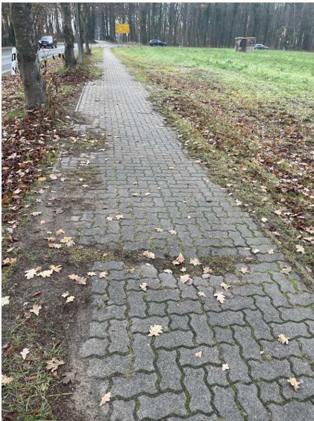
Foto 04: Station ca 0+85,00 in Richtung B111
